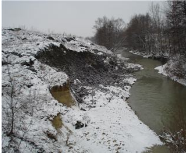
Figure 7. Reforestation may be more reliable than other engineering works – e.g. Panga Nord coal mining tailing waste deposit landslide, Vâlcea County.
