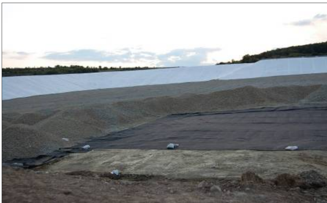
Figure 8. Installation of the waterproofing system at Dumitra-Tărpiu.
