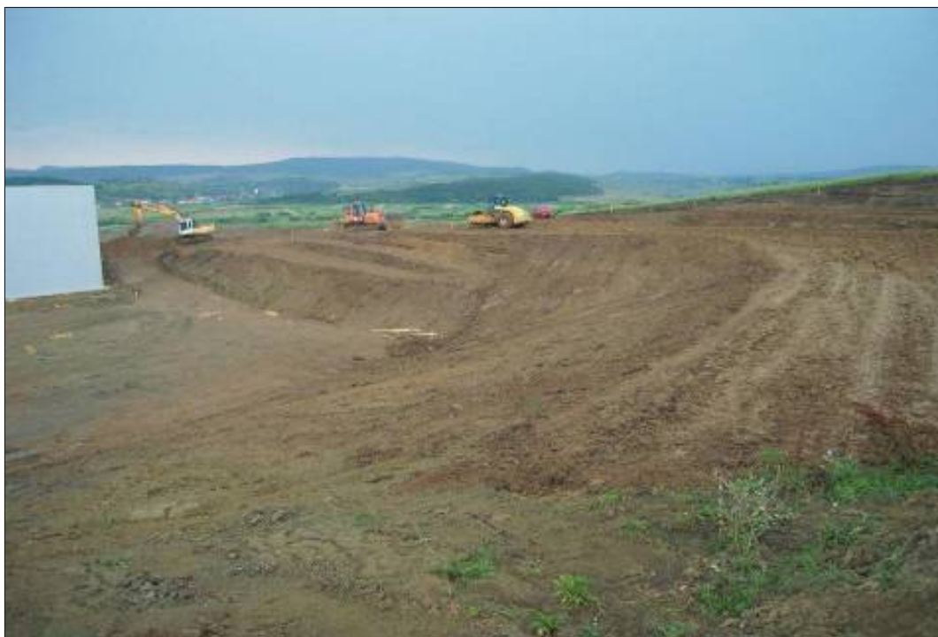
Figure 7. Slope repair between road DA2 and the plastic materials storage-platform.
