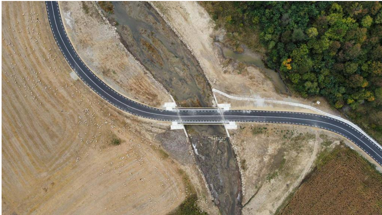
Figure 3. The new bridge over the Șieu River (source: https://rasunetul.ro ).
